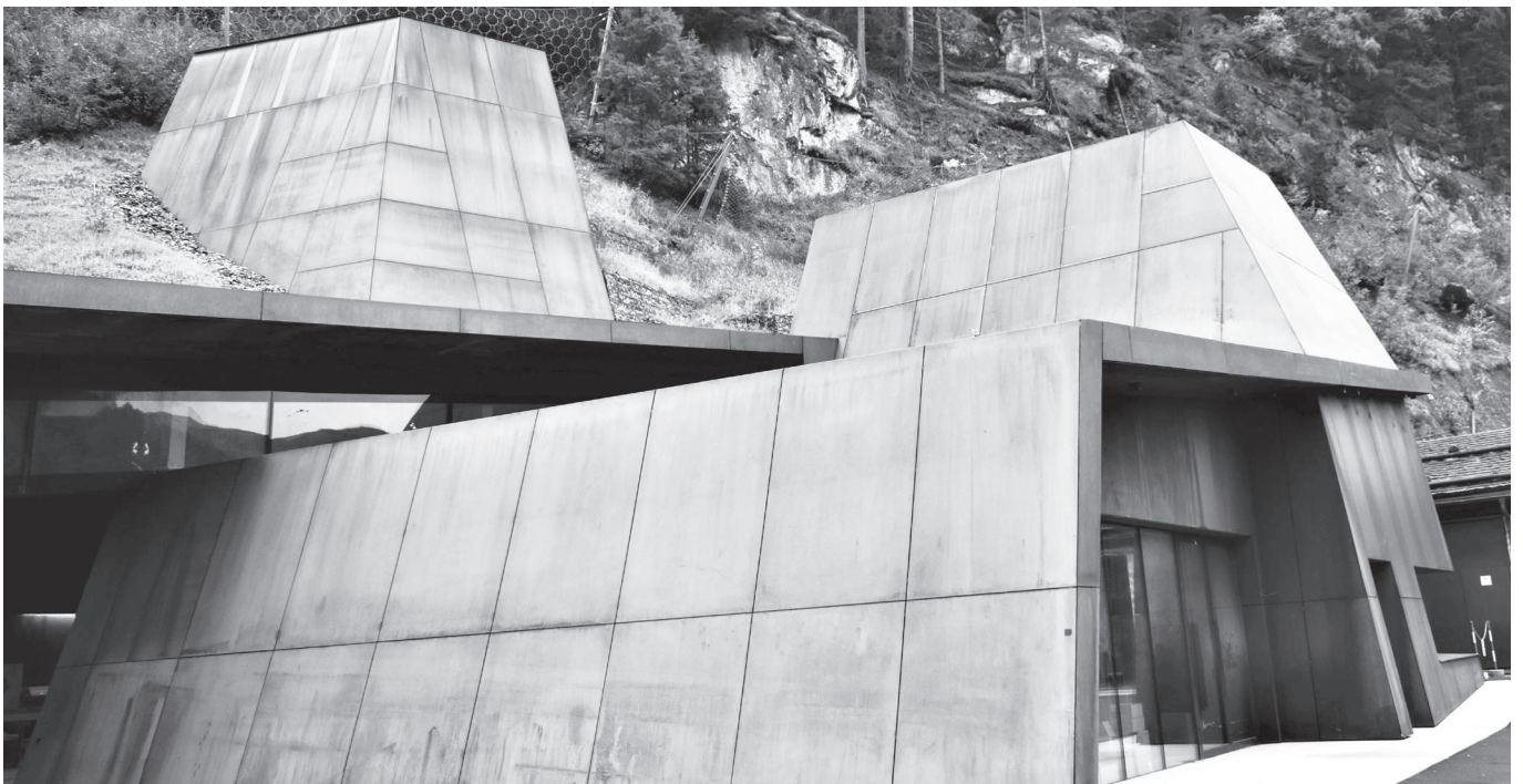
Musealer Zubau - Remise
